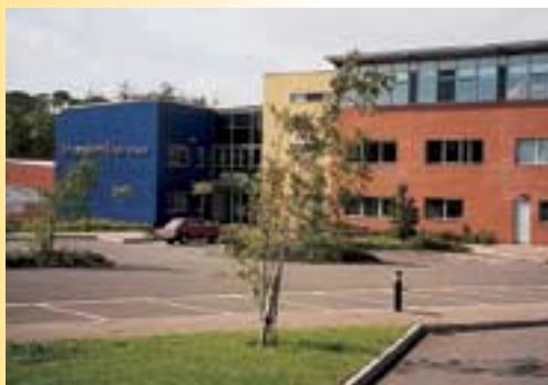
Figure 1.22 Drumglass High School, Dungannon
